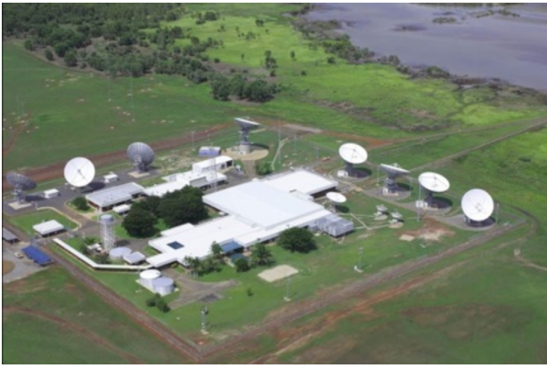
Shoal Bay Receiving Station, January 2013
