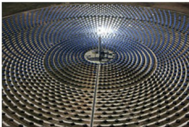
Fig. 7. Gemasolar power tower plant in Spain
