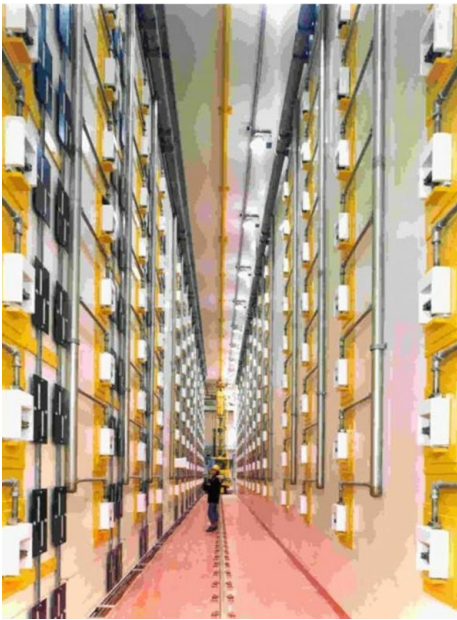
Plutonium storage area, Sellafield, England
