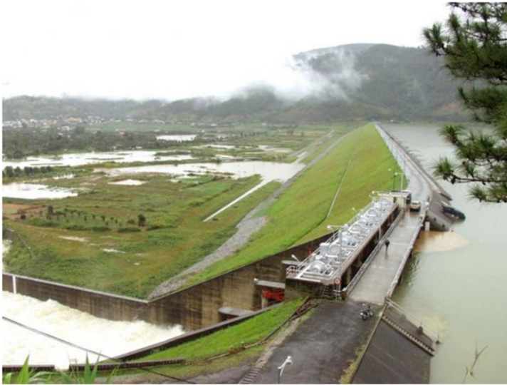
Da Nhim flood control gate
