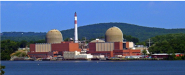
Indian Point Nuclear Power Plant
