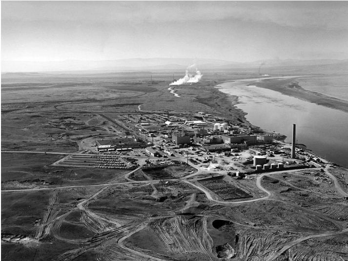
Hanford reactors along the Columbia River, 1960
