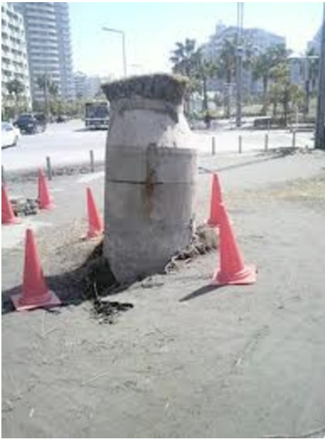
“Manhole Tower”, Urayasu, Chiba
