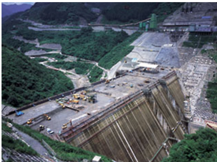
Takizawa Dam, second construction
