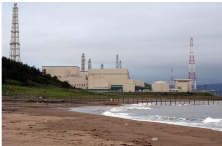
The Kashiwazaki-Kariwa nuclear power plant.
