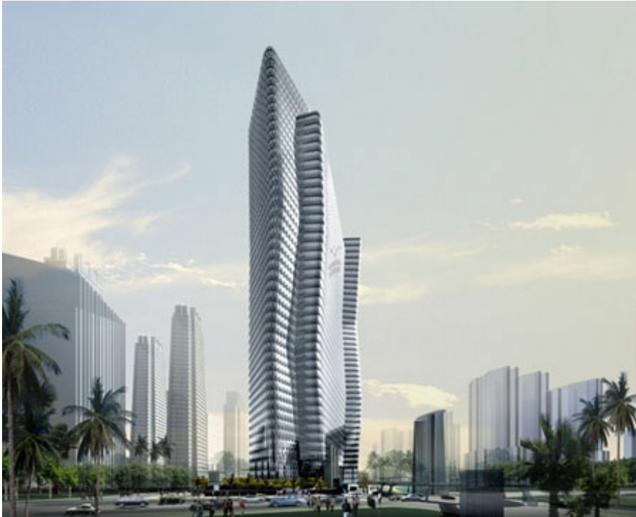
Bakri Tower, Jakarta
