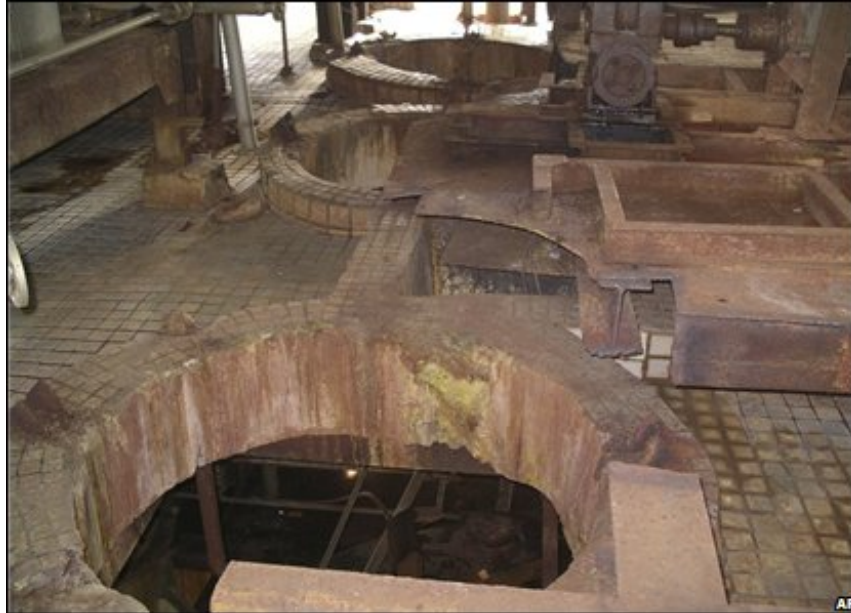
Pyongyang agreed to close the reactor and remove fuel rods
