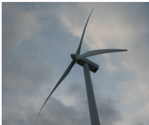
Yokohama's wind turbine
