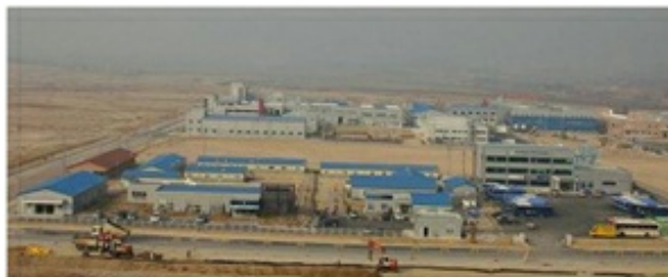
<Gaeseong Industrial Complex>
