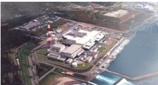
The Kashiwazaki nuclear power plant
