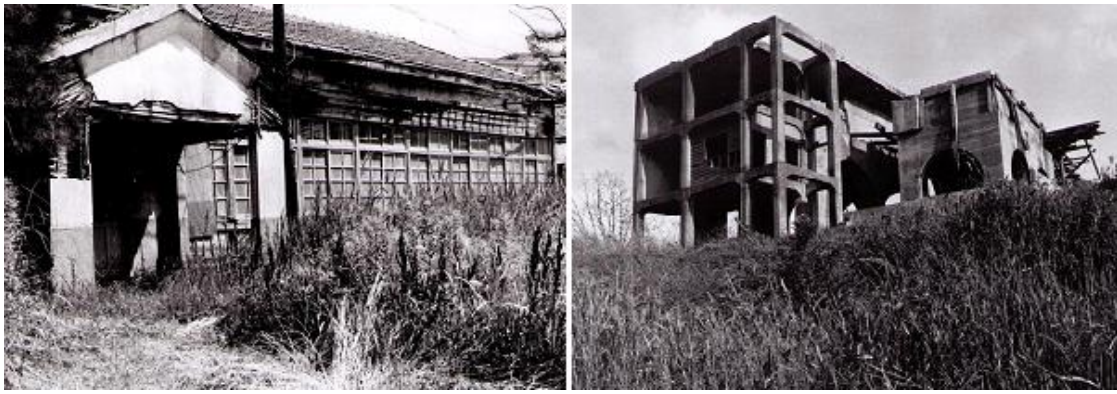
The abandoned Aso Yoshikuma work office (left) and ruined Yoshikuma mine buildings in the late 1970s. (Hayashi Eidai photos)
