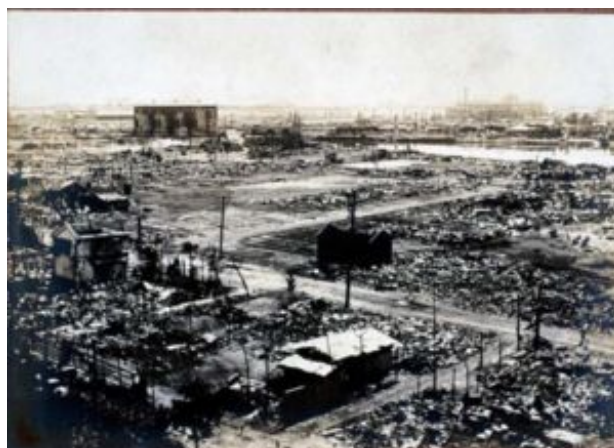
Earthquake destruction in Yokohama
