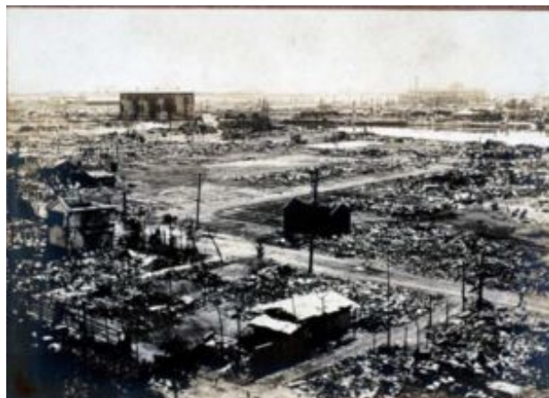
Earthquake destruction in Yokohama
