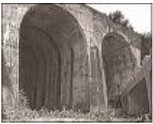
The bridge at No Gun Ri
