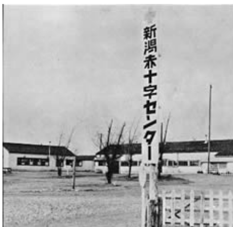
Japan Red Cross Center in Niigata
