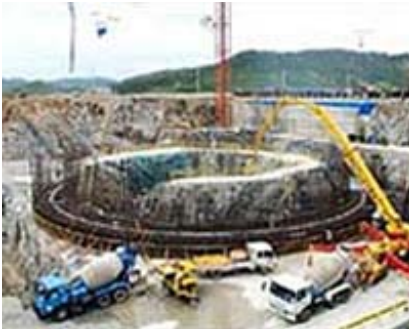
Incomplete light water reactor in North Korea
