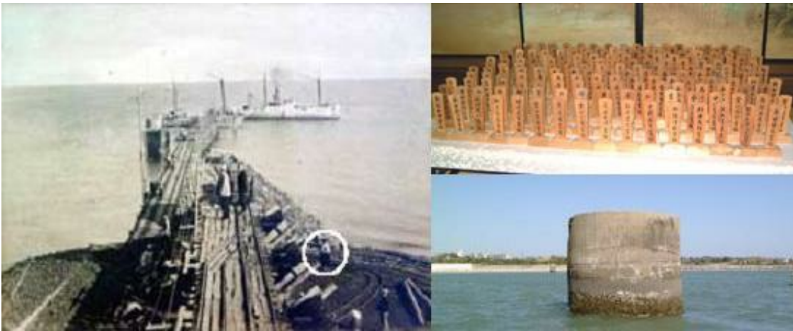
Chosei Mining's undersea mine near Ube city, concrete ventilation shaft, and Korean mortuary tablets (photos by Chosei Tanko "Mizuhijo" Historical Preservation Group)
