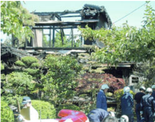
The frame of the Kato home following the fire
