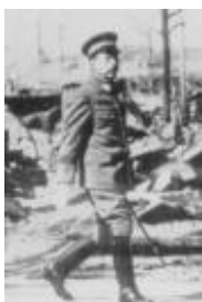
Hirohito inspects bombing damage on the verge of Japan's surrender
