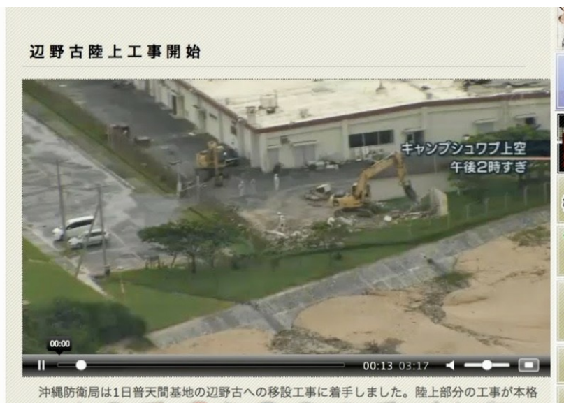
Image 1. Henoko construction started: TV clip from QAB Asahi
